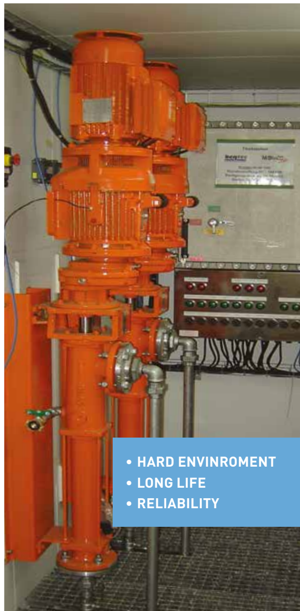
Oil drilling plant: speed variators on screw pumps (Atex ambient)
